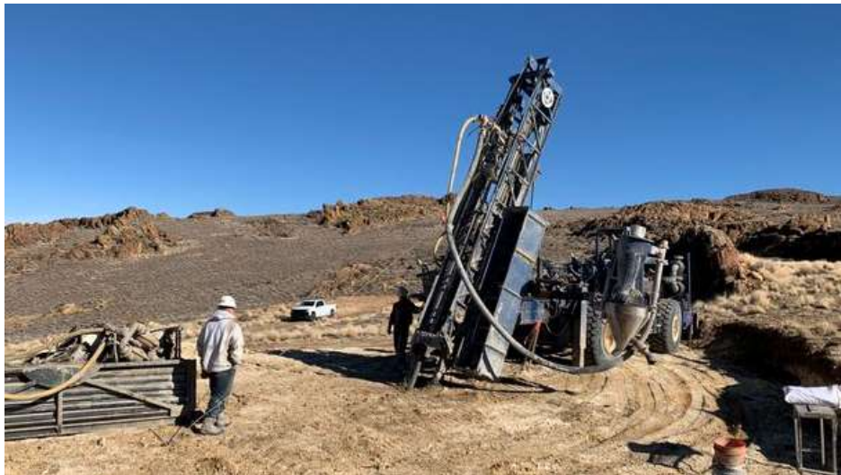
Figure 4: Drilling at Airport
