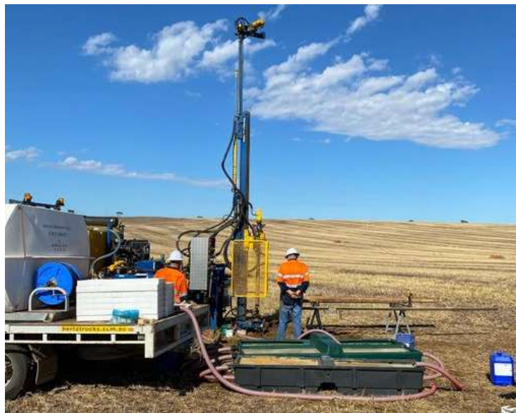
Figure 2: Geotechnical drilling for the plant and TSF at Hillside
