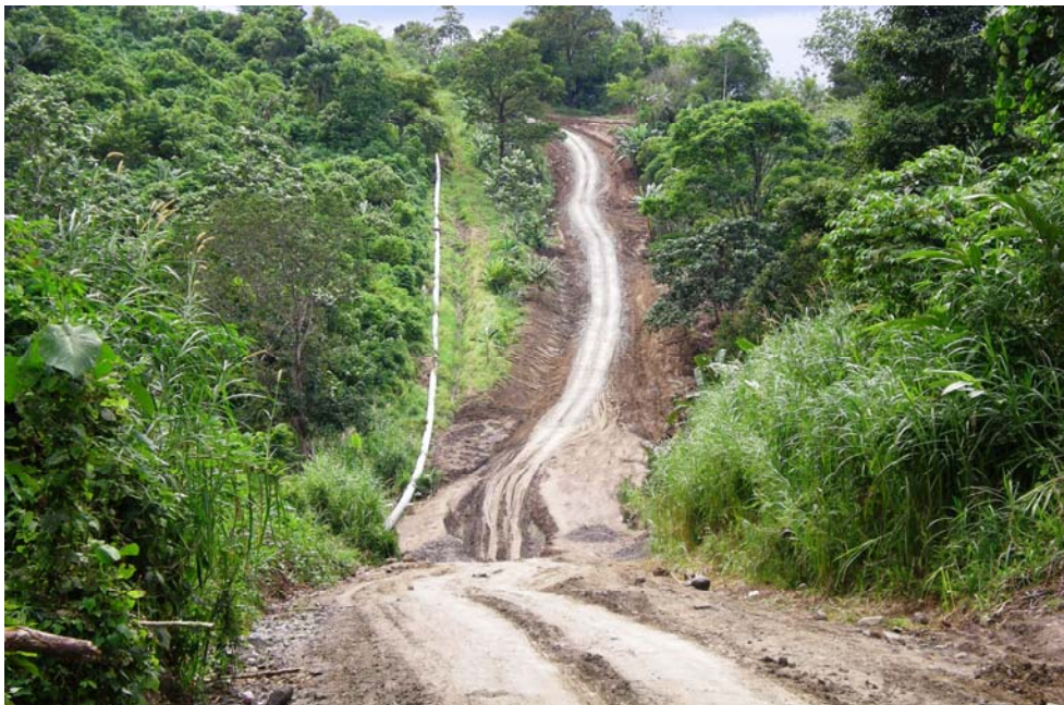
Figure 3 Ramu Pipeline Crosses A Steep Valley
