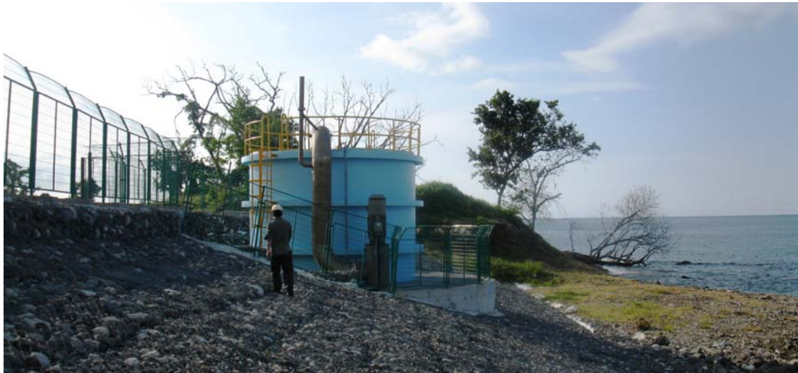
Figure 7 Tank Mixing Tailings with Seawater
